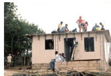
Habitat home being built in Jamaica.
