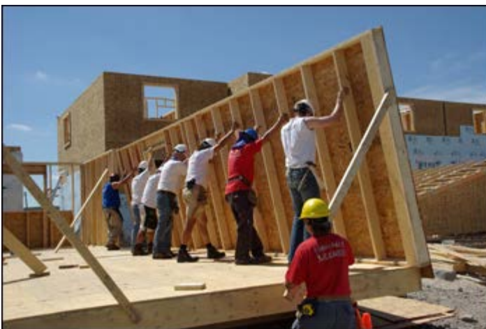
The essence of team work as volunteers raise a wall together.
