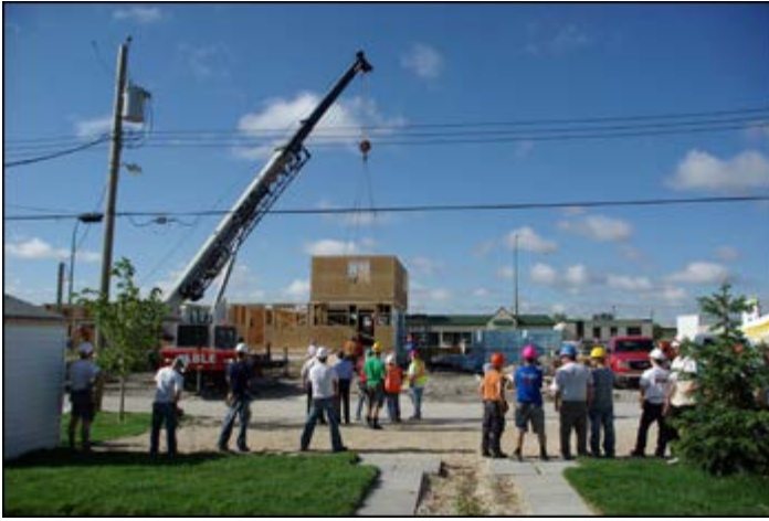
Raising the second floor of a side-by side in perfect position.
